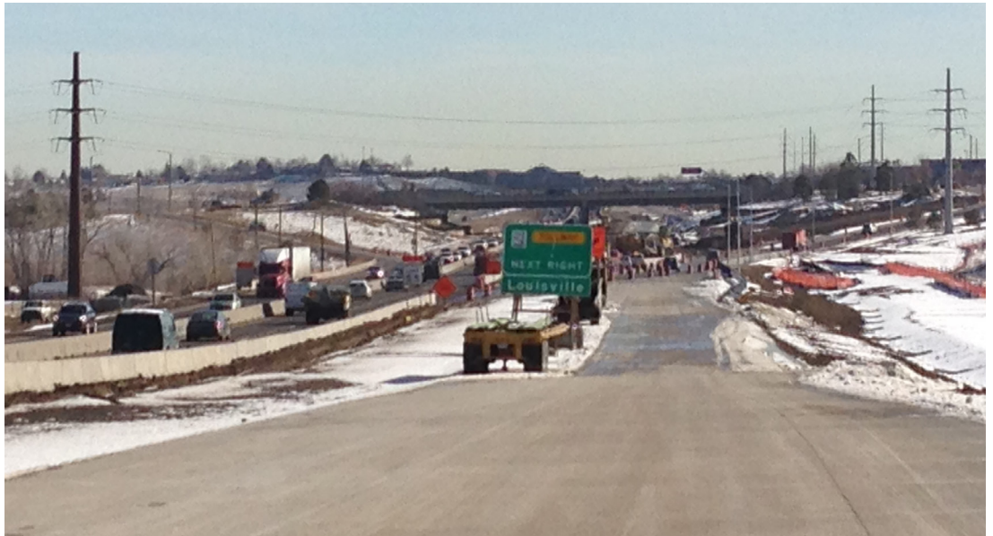
Permanent concrete paving on eastbound US 36 at Interlocken
